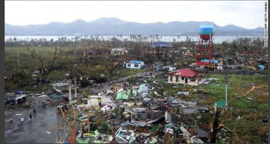
Houses are destroyed by the strong winds caused by the typhoon in Tacloban City.
