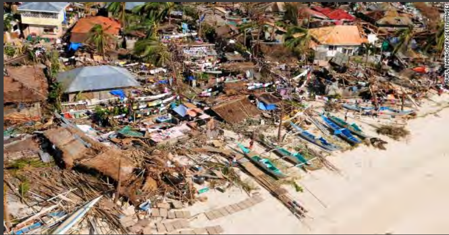
Devastation is everywhere in Iloilo in the aftermath of the typhoon.
